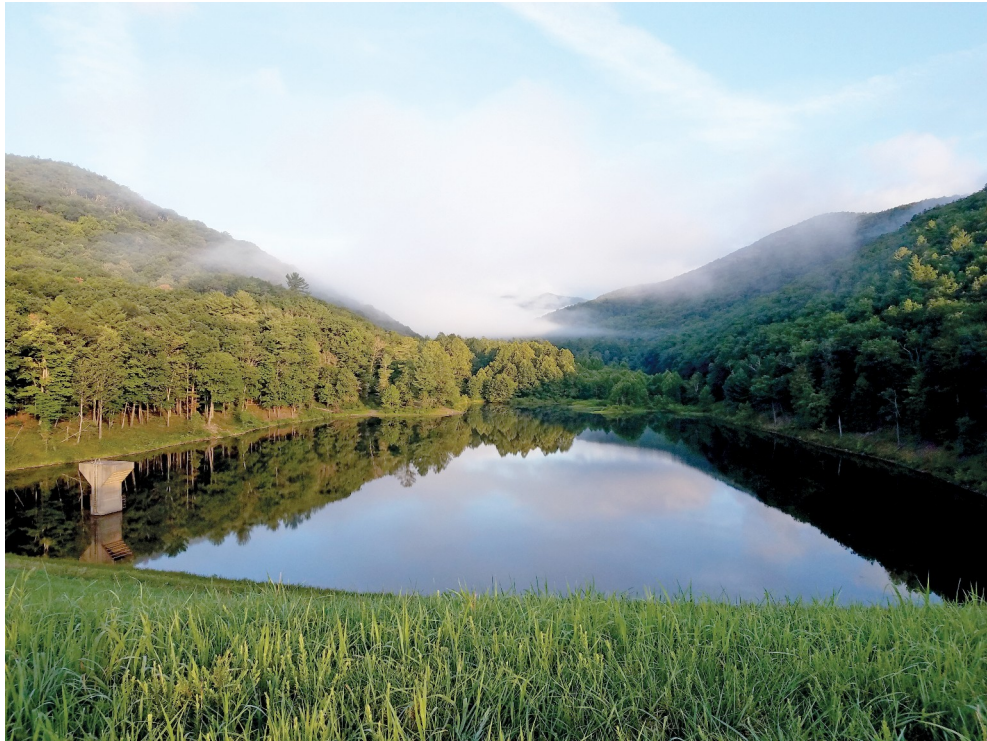
Hearthstone Lake Dam located in Augusta County, Virginia
